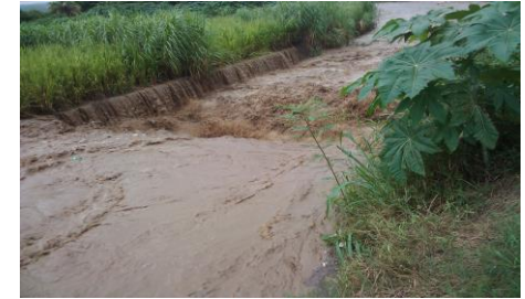
1] San Juan River – Weir, Irrigation System, Stilling Basin, Sedimentation Basin
